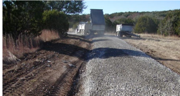
Laying down aggregate road base
