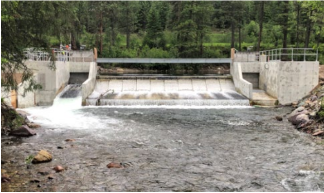
Jocko K Diversion and Fish Screen at Flathead Indian Irrigation Project (FIIP), Montana.
