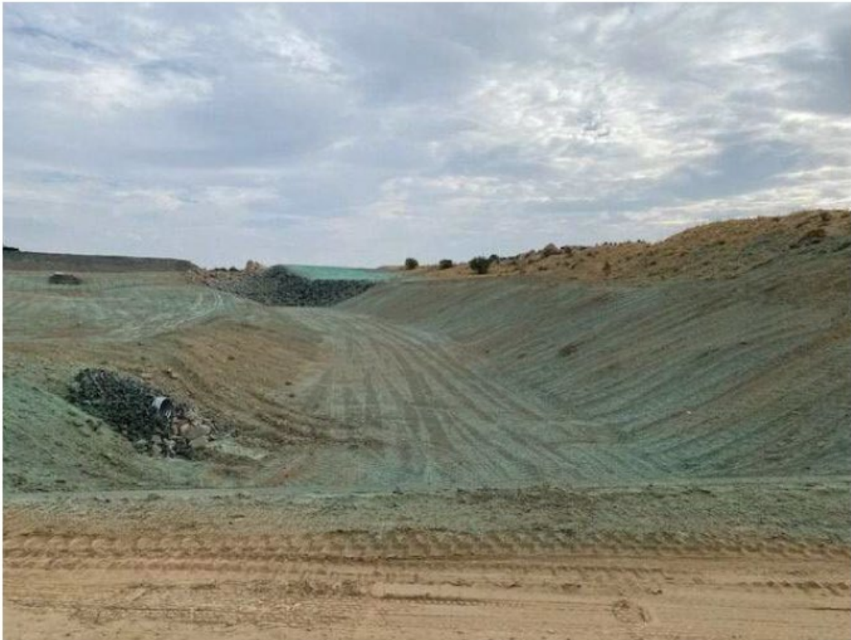
To'hajiilee Dam Spillway, August 2023
