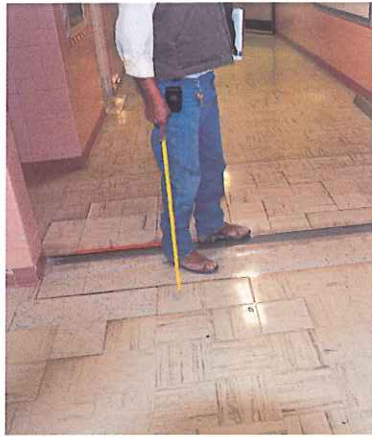
Location: Elementary School Building 431 Backlog No.: N36-08-431-X-001-1 Deficiency: Vinyl Asbestos Tiles flooring, cracking , popping up throughout interior of building
