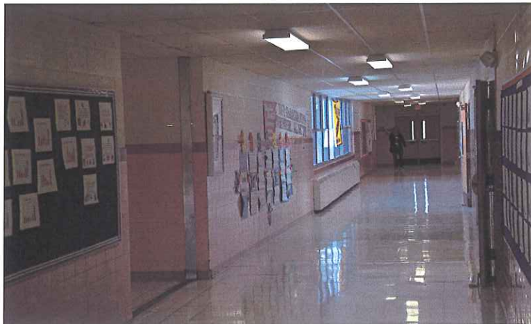
Location: Elementary School Building 431 Backlog No.: N36-08-431-M-022-1 Deficiency: Upgrade electrical including lighting, fire alarm, and telecommunication.
