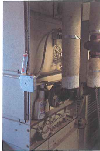
Location: Cafeteria/Dining Hall Building 434 Backlog No.: N36-08-434-M-036-1 Deficiency: Boilers for hydronic heating systems are in poor condition with only minimal temperature controls
