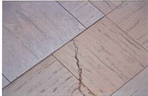
Location: Elementary School Building 431 Backlog No.: N36-08-431-X-001-1 Deficiency: Vinyl Asbestos Tiles flooring, cracking , popping up throughout interior of building
