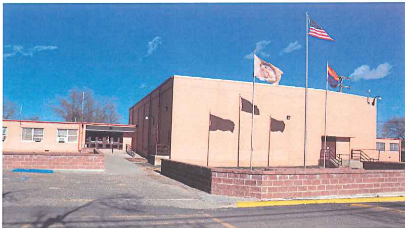
Location: Elementary School Building 431 Backlog No.: N36-08-431-F-006-2 Deficiency: Upgrade building fire alarm and tie in to other facilities with fiber optic lines.
