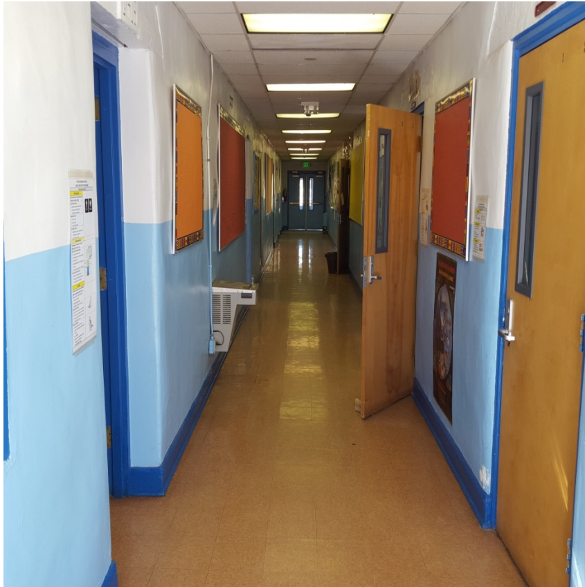
A Hallway to go From Room to Room Without Exposure to the Elements
