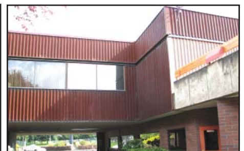
Additional insulation could be installed if this badly deteriorated steel siding is replaced with new low maintenance, pre-finished material.
