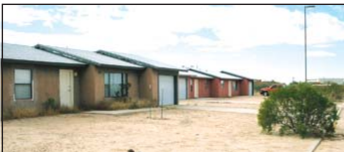
Employee housing at Tohono O'odham High School in Arizona.
