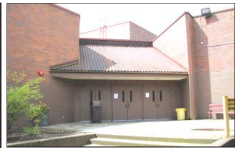
Installing weather stripping, astragals and door sweeps on these exterior doors will eliminate drafts and dust. (Red shows heat loss).
