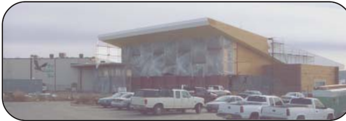
The new gym is being built next to the old gym.
