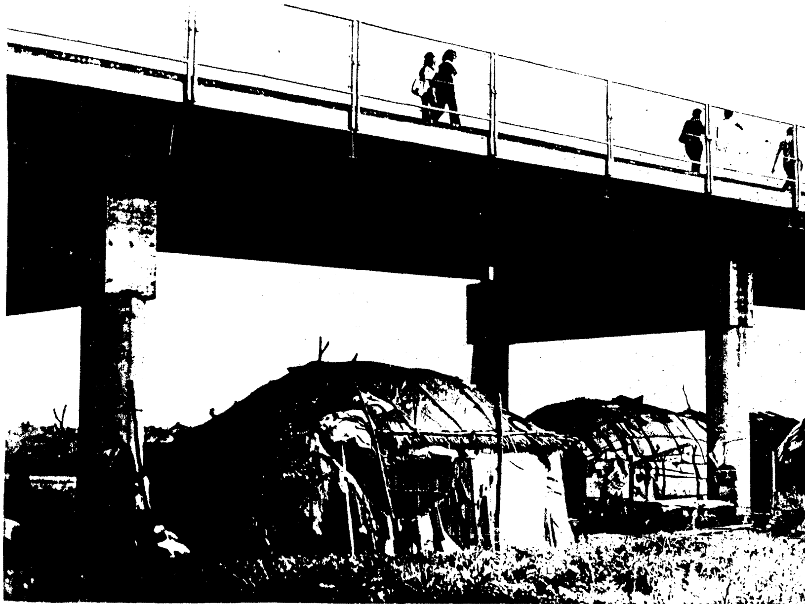
Kickapoo Housing Conditions under the International Bridge in the Flood Plain of the Rio Grande River at Eagle Pass.
