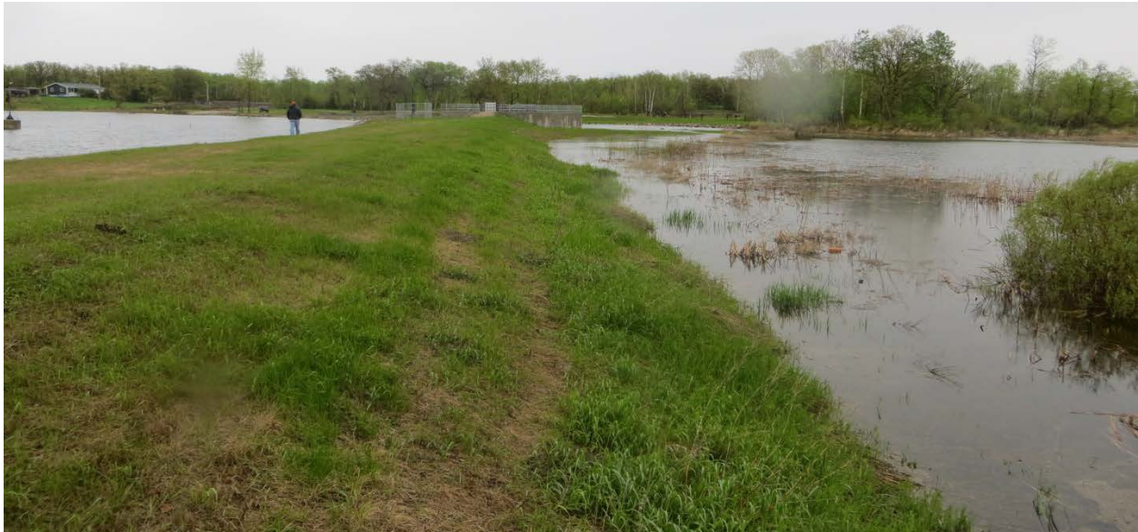
Belcourt Dam, ND
