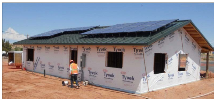
PS&J Quarters under construction in Moencopi, Arizona
