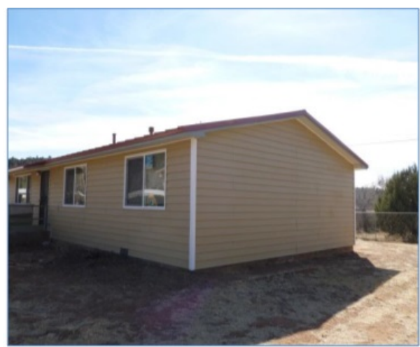
After – Renovated quarters with new siding, windows and roof
