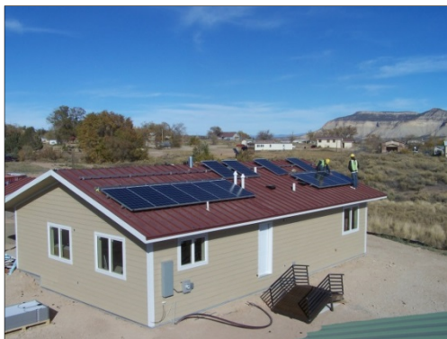
PS&J Quarters under construction near Ute Mountain in Colorado
