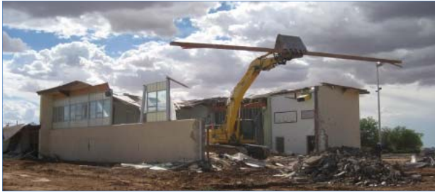
Demolition of an old Library at Dilcon Community School in Arizona.
